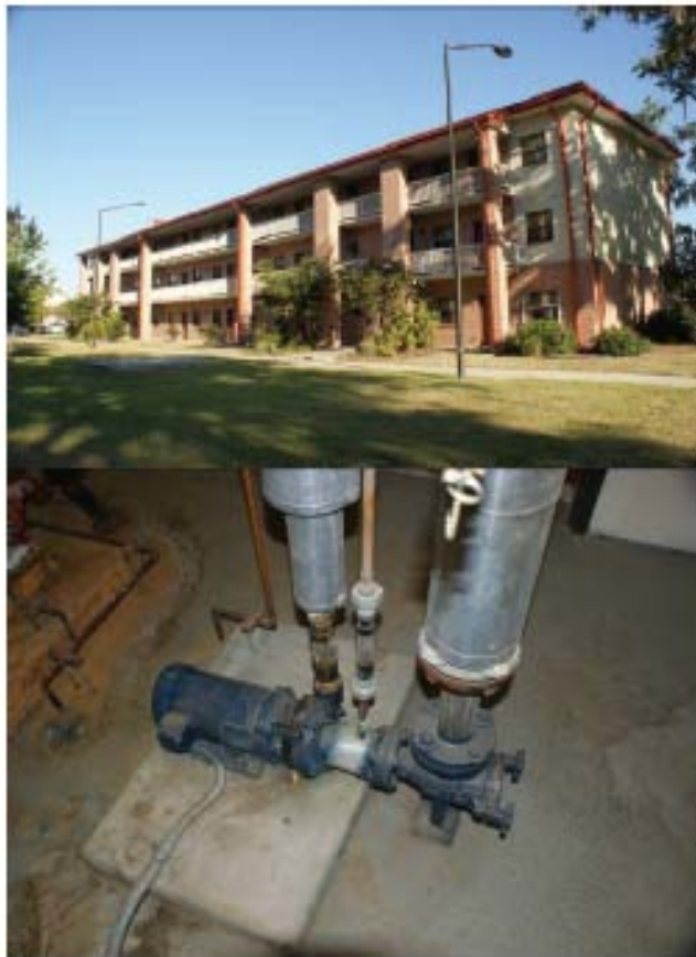
Barracks 1511 - 3HP Constant Speed End Suction Pump
